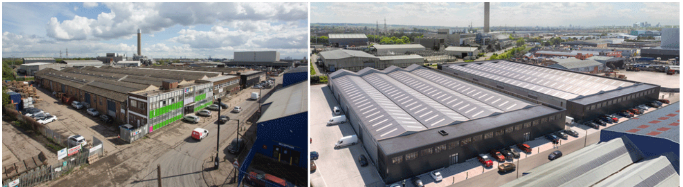
Edmonton Industrial Park before and after development
